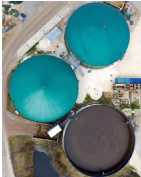
Biogasanlage Foto: iStockphoto.com/Bim
